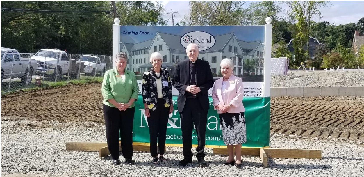
(l. to r.) Sr. Kay Ryan, CSJ, Sister Charla Commins, CSJ, The Most Reverend Howard J. Hubbard, Bishop Emeritus, and Sr. Lauren VanDermark, CSJ pose in front of the construction site of Shaker Pointe's new building, Parkland at Shaker Pointe, which will offer rental opportunities for residents.
