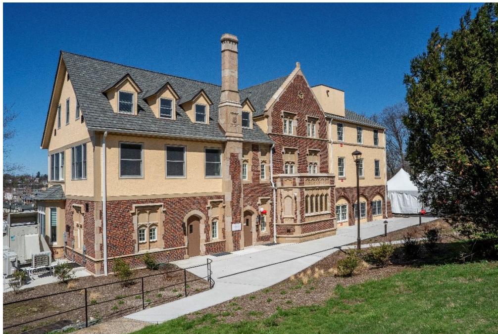
Once an abandoned convent, now the new St. Frances Cabrini Apartments will be a home to young neurodiverse adults.
